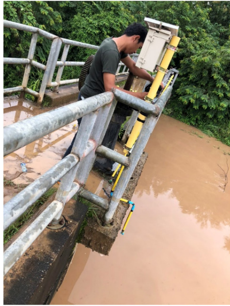
(b) Automatic water level gauges at Pua river outlet
